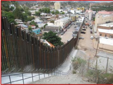
Nogales, Ariz., Border Fence Replacement
