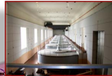
Bull Shoals Powerhouse Arkansas
