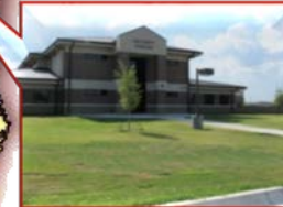
Little Rock AFB Security Forces Operations Facility
